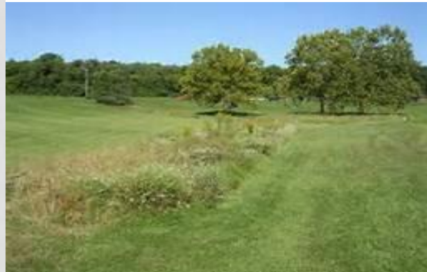
Figure 5. Swale at I-4 Maitland Interchange-East.
